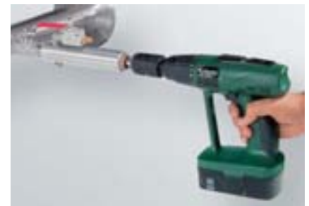
Drilling under pressure
